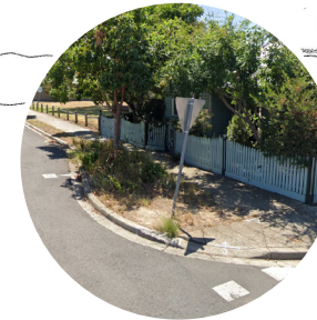
No. 85 Coronation Street frontage (Existing Condition)
