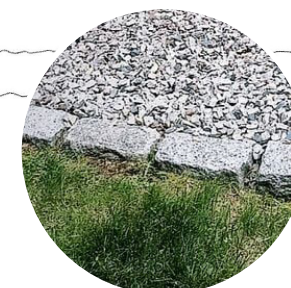
Bluestone pitch edging and decorative pavement
