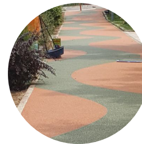
Coloured concrete to convey restricted vehicle zone with pedestrian priority
