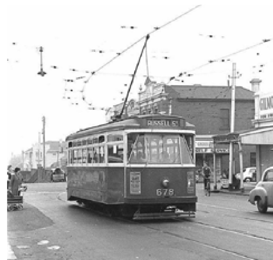
Victoria Street Tram - https://www.seddon-village.com.au
