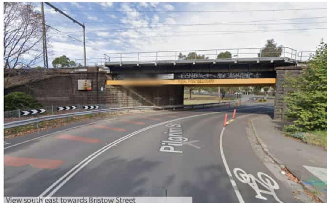
View south east towards Bristow Street
