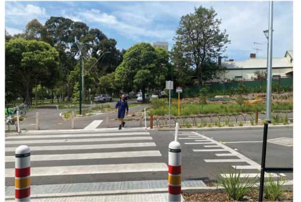
WSUD interventions and improved pedestrian priority, South Kensington Station
